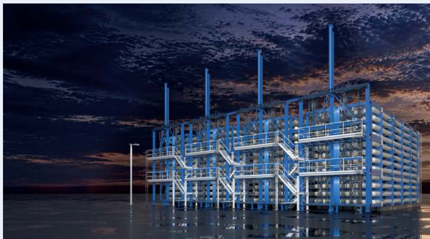
Visualisation of a plant concept with four storage blocks of six modules each.
